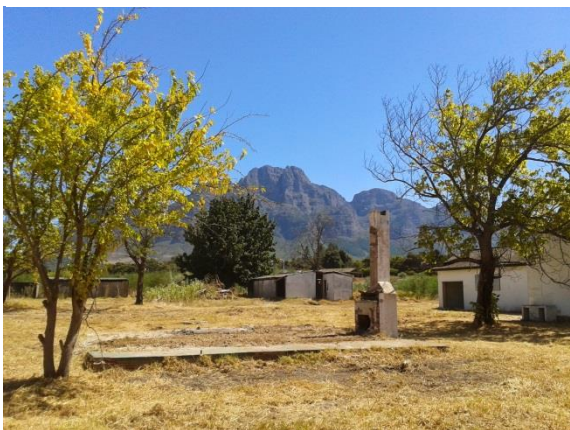
Figure 8. Uninhabited cottages (one demolished) in Section C
