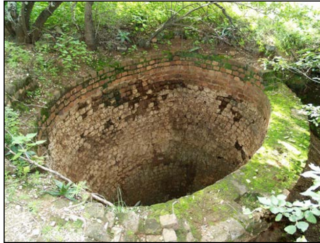
Figure 27: One of the lime kilns near the Sterkfontein Country Estate in the WHS
