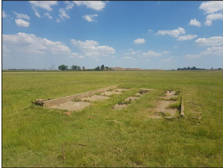
Figure 5-1: A concrete floor structure dating to the Historical Period at Site Exigo-NGP-HP01.
