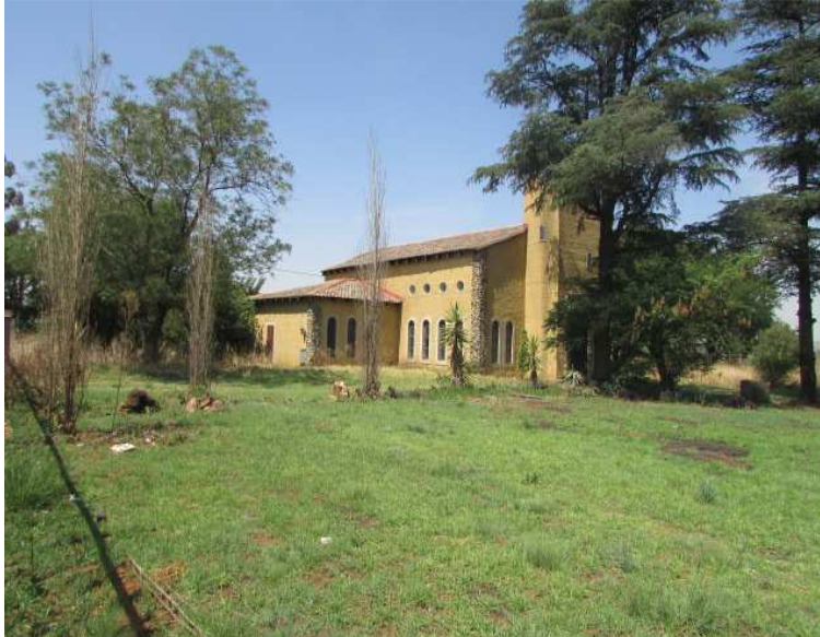
Fig.10: A view of the existing Wedding Chapel on the Antiqua site.
