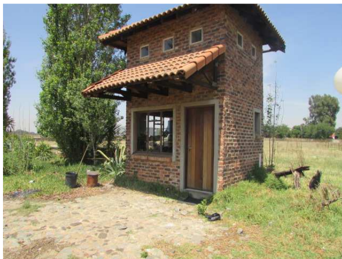
Fig.20: The Security building here.
