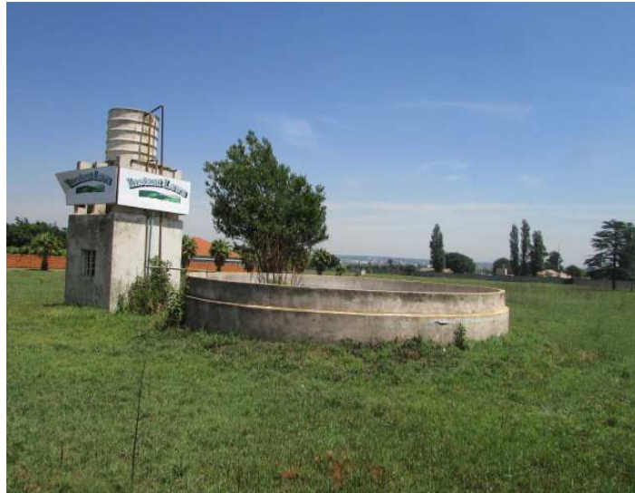
Fig.23: The cement dam and water tower in the Proposed New Cemetery area.
