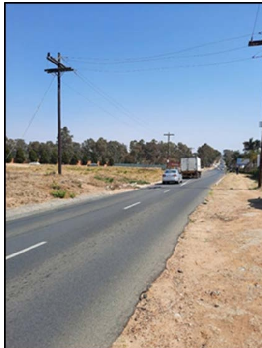
Figure 3.6. General site conditions - Network 3 alternate route.
