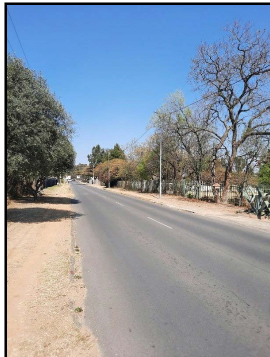
Figure 3.4. General site conditions - Network 1 alternate route.
