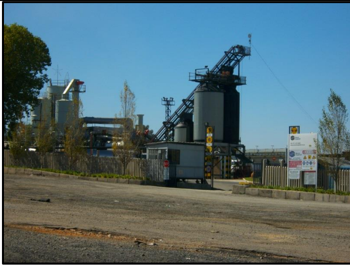
Figure 13: Much Asphalt viewed from the West.
