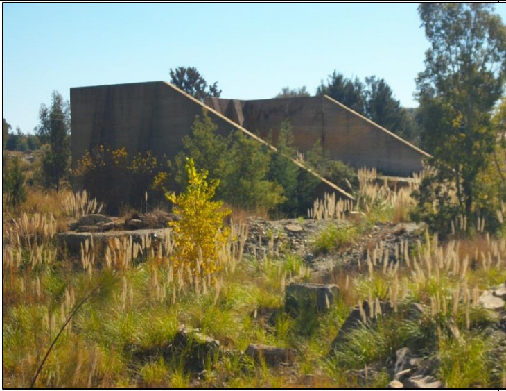
Figure 20. Southern view of reduction works and demolished structures.
