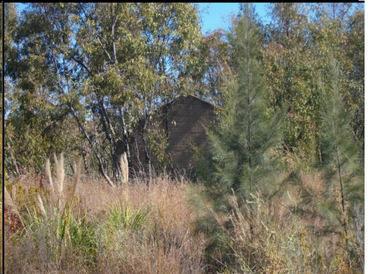
Figure 23. Ruin 2 made from cement bricks.
