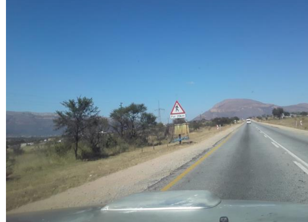
Figure 35: View of the R37 route to where the pipeline will pass through
