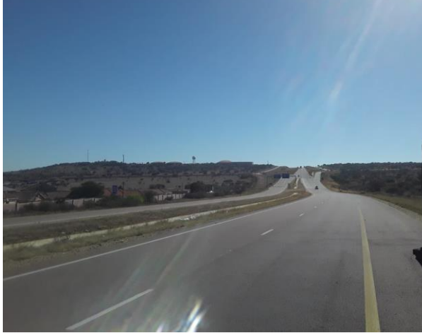
Figure 34: View of the R 37 Route
