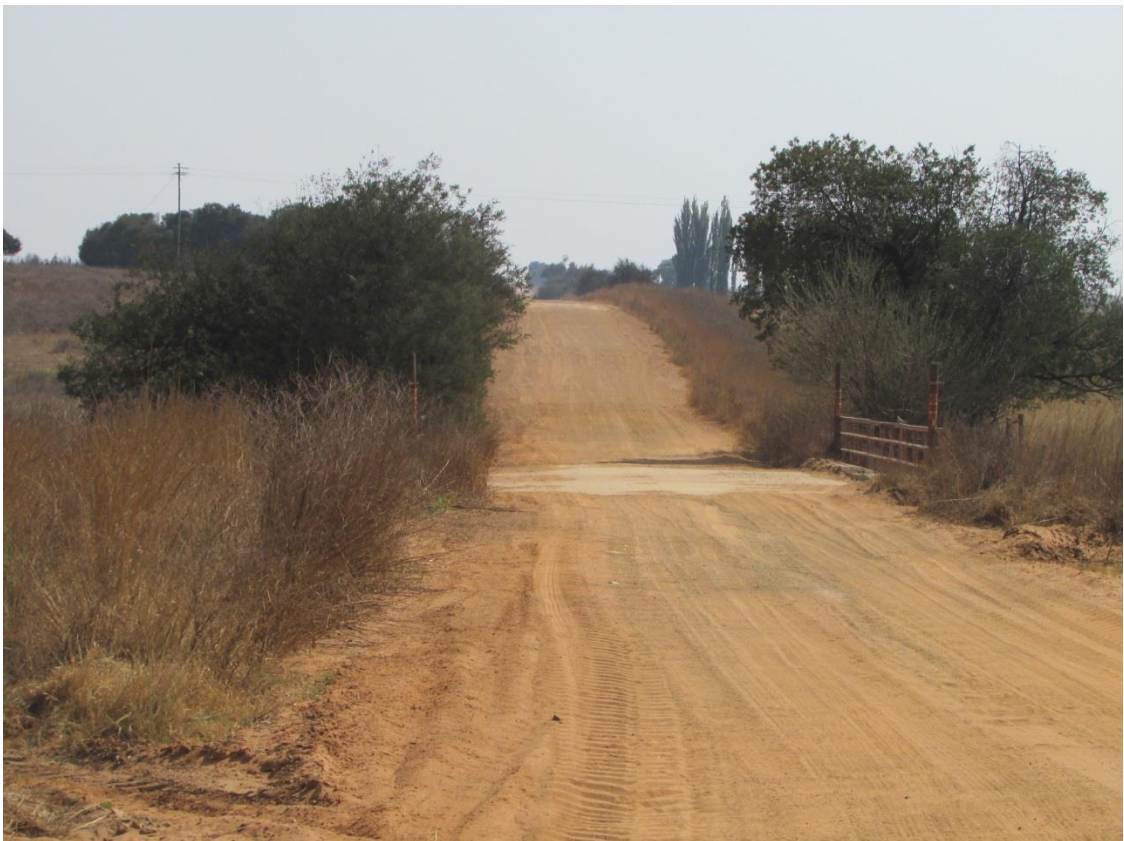
Figure 18: A section of Pipeline Route 2 at a stream crossing.
