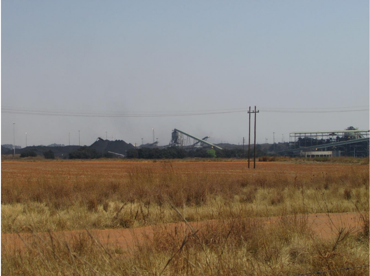
Figure 20: A view towards the mining area in the north where Route 2 and Route 3 junctions.
