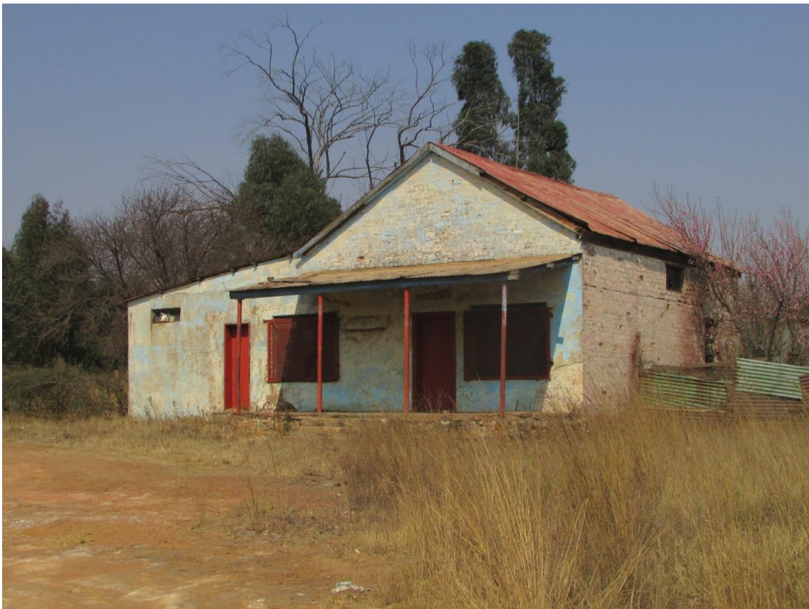
Figure 16: One of the old structures (Site 1) close to Pipeline Route 2.
