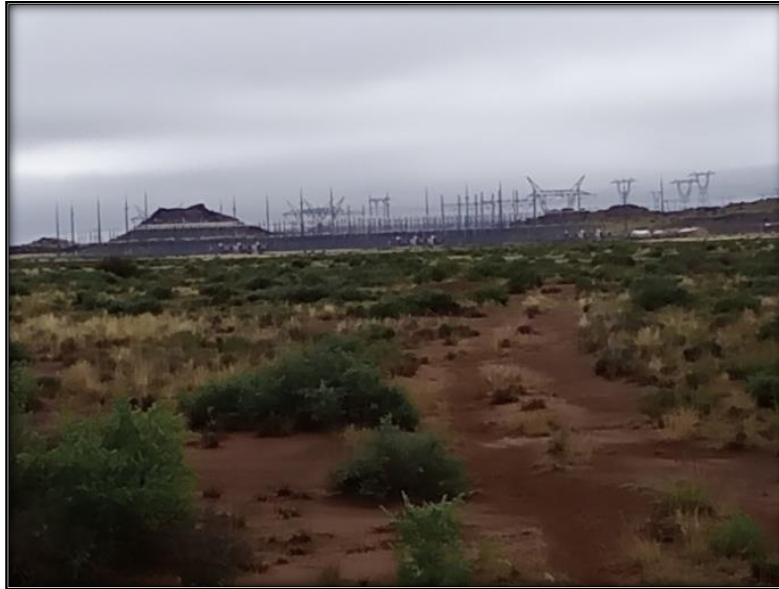
Figure 12: View over Gamma Substation
