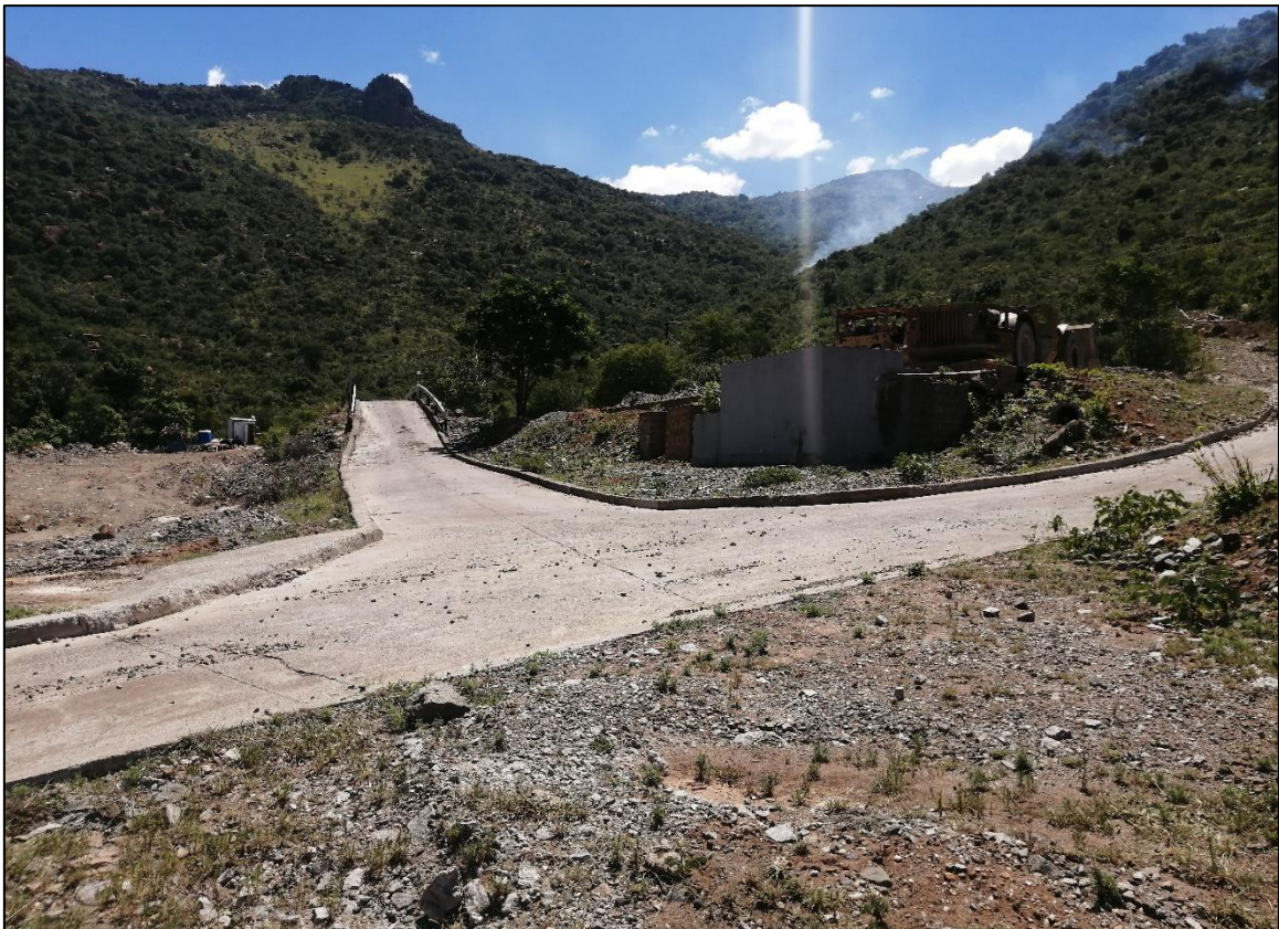
Figure 8 – View of existing mining infrastructure located within the study area.
