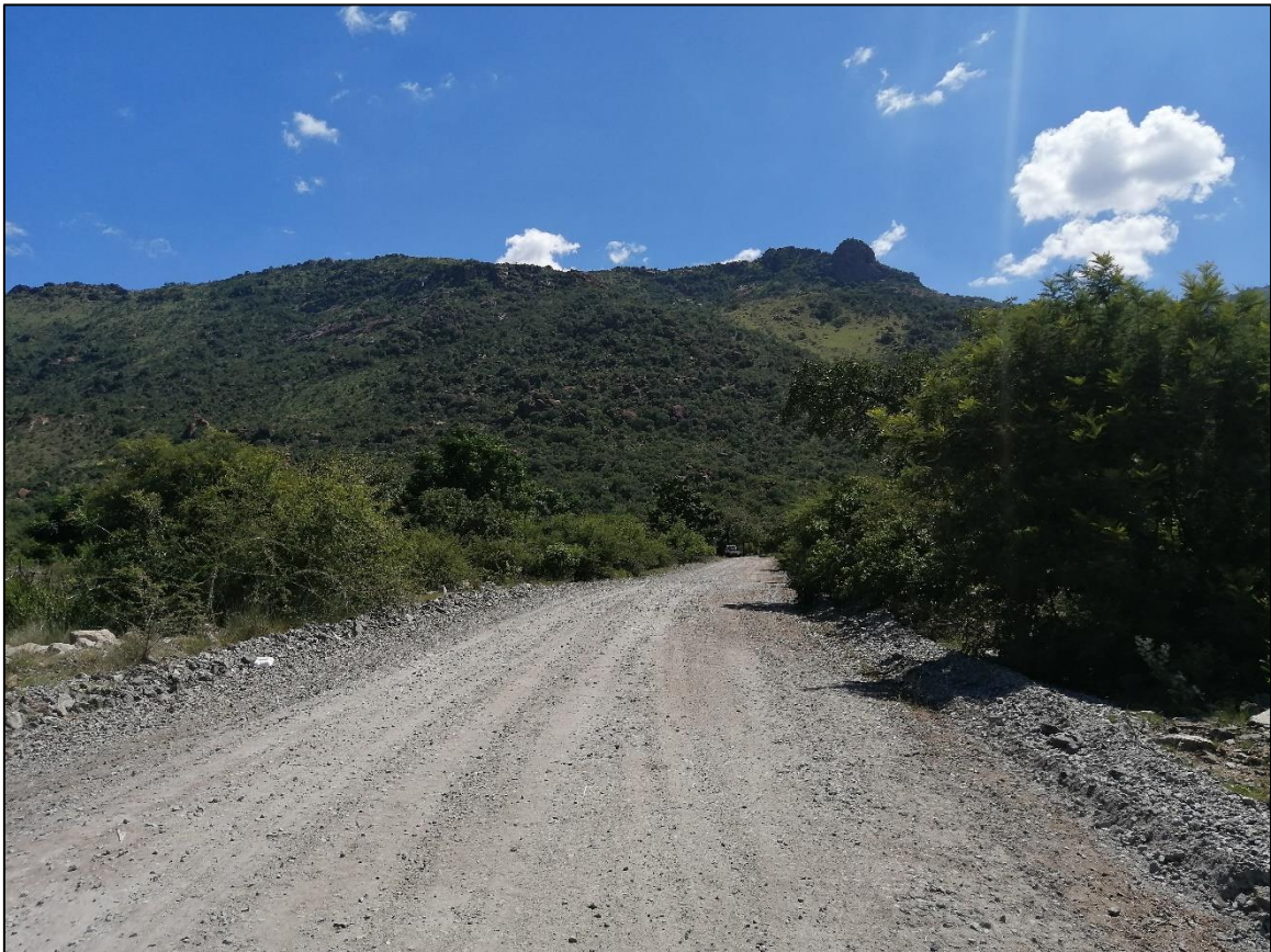
Figure 6 – Another view of the study area, showing a section of the existing road.
