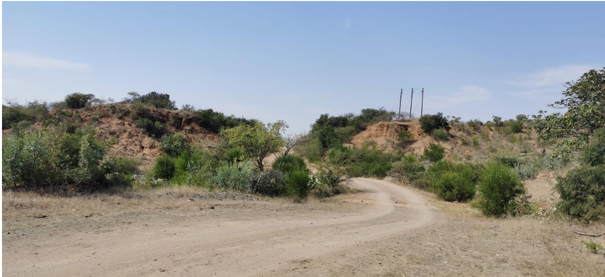
Figure 11 - View of the northern access road area
