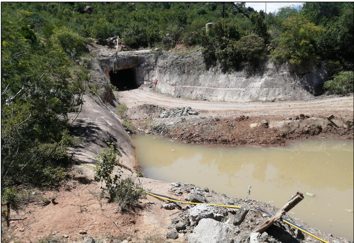
Figure 10 - View of another mine adit from within the study area. This adit is reinforced with concrete and appears to be still in use today.
