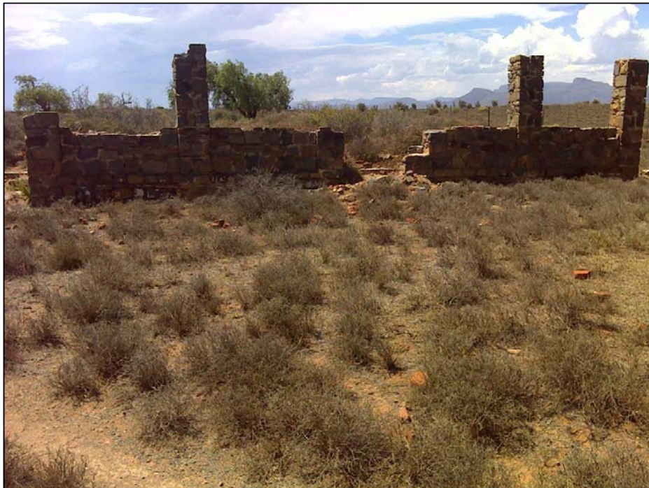
Figure 34. View of the remains of the dwelling.
