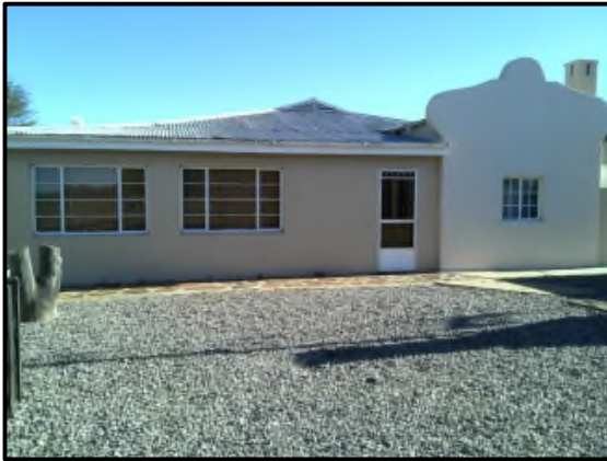
Figure 7: Farmhouse at Site 3.
