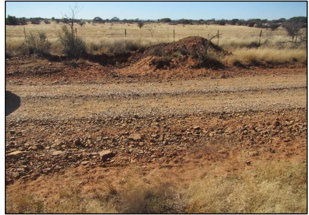
Figure 8: View across road to be upgraded looking towards the northeast.
