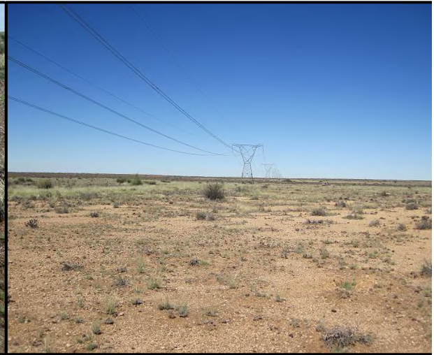
Figure 6. Existing powerlines (Aries/Helios 1 400kV).
