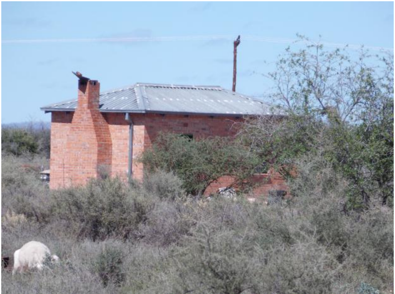
Figure 4. Labour housing on site
