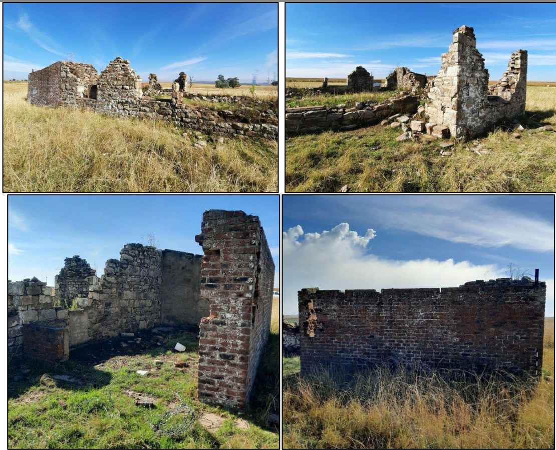
Figure 20: Stone farmhouse ruin with brick garage addition.
