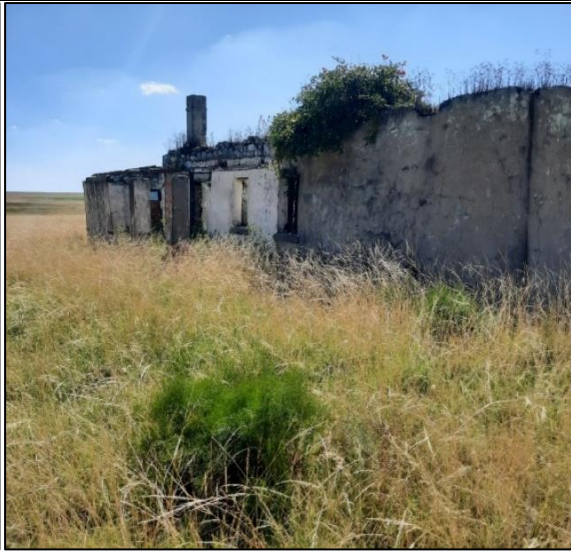
Figure 28: A cement and stone house ruin.
