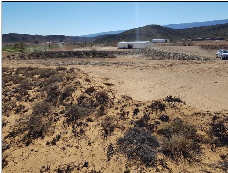
Figure 3-10: View of general surroundings at the site of the newly constructed dam subject to the S24G rectification .
