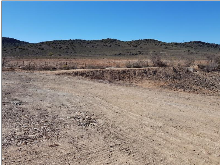
Figure 3-4: View of general surroundings at the site of the newly constructed dam subject to the S24G rectification
