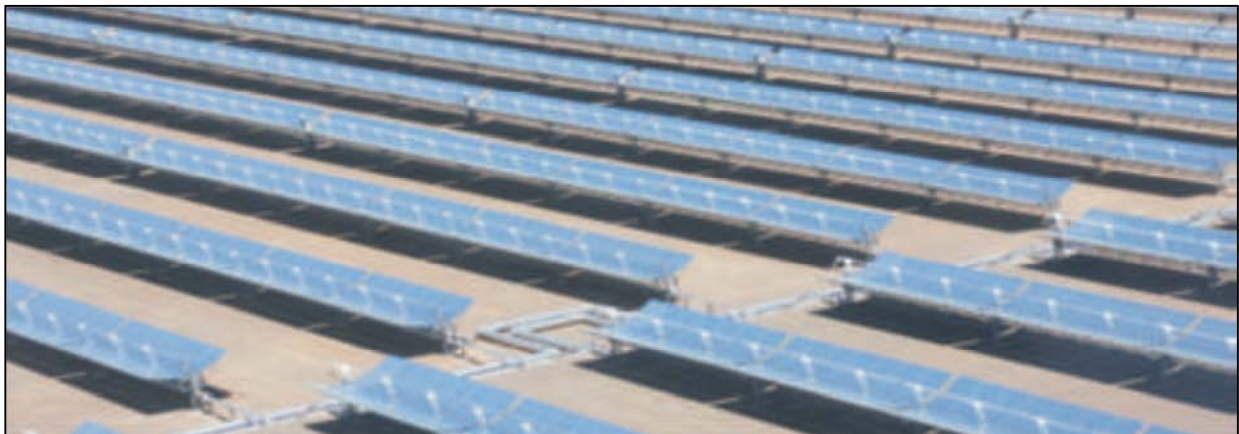
Figure 3. Example of reflective solar plants (parabolic troughs).
