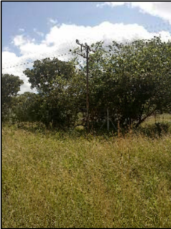
Figure 7-7. Overgrown vegetation and power lines running next to the road.
