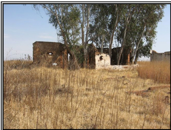
Figure 11-2: Remains of the old Structures on site (PGS, 2009)
