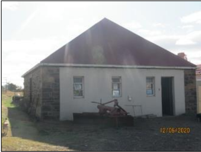
Figure 33 - View of the garage located next to the main farmhouse.
