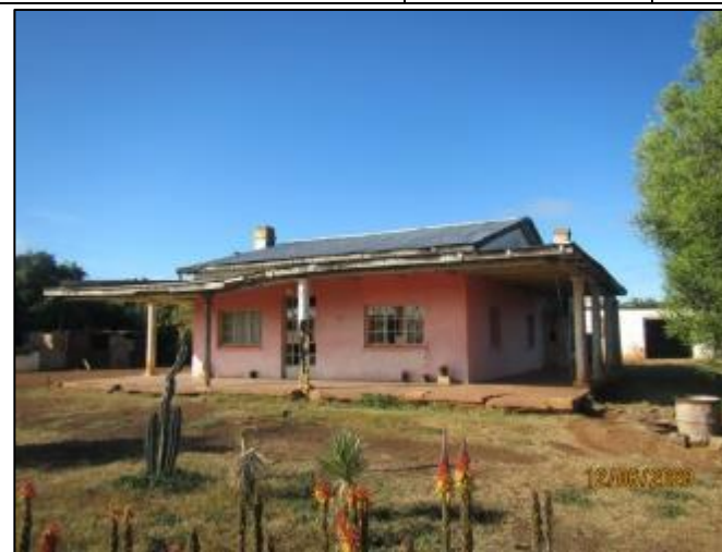
Figure 24 - View of the northern façade.
