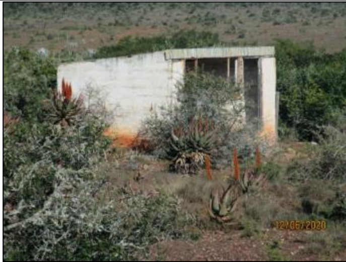
Figure 25 - View of the outbuilding.
