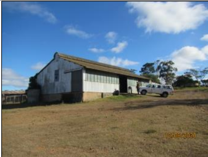
Figure 37 - View of the bigger shed.
