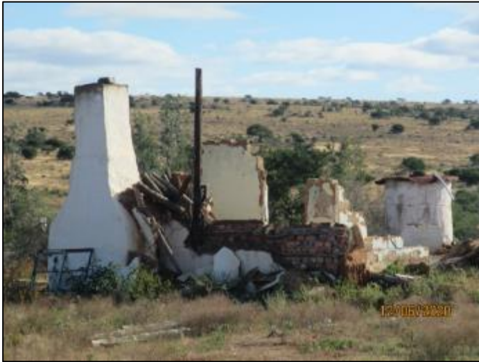
Figure 45 - Demolished labourer house.
