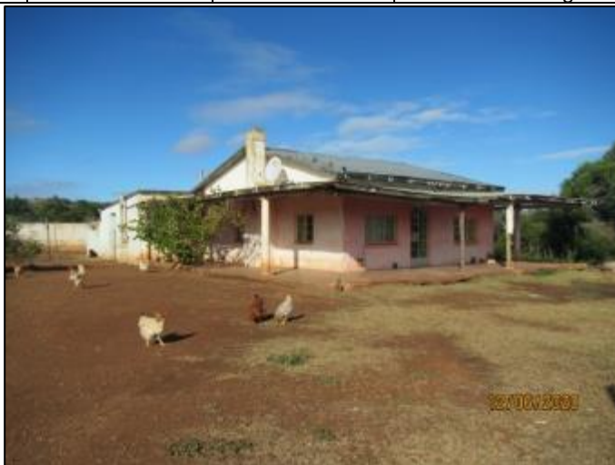
Figure 23 - View of the north-eastern corner of the house.
