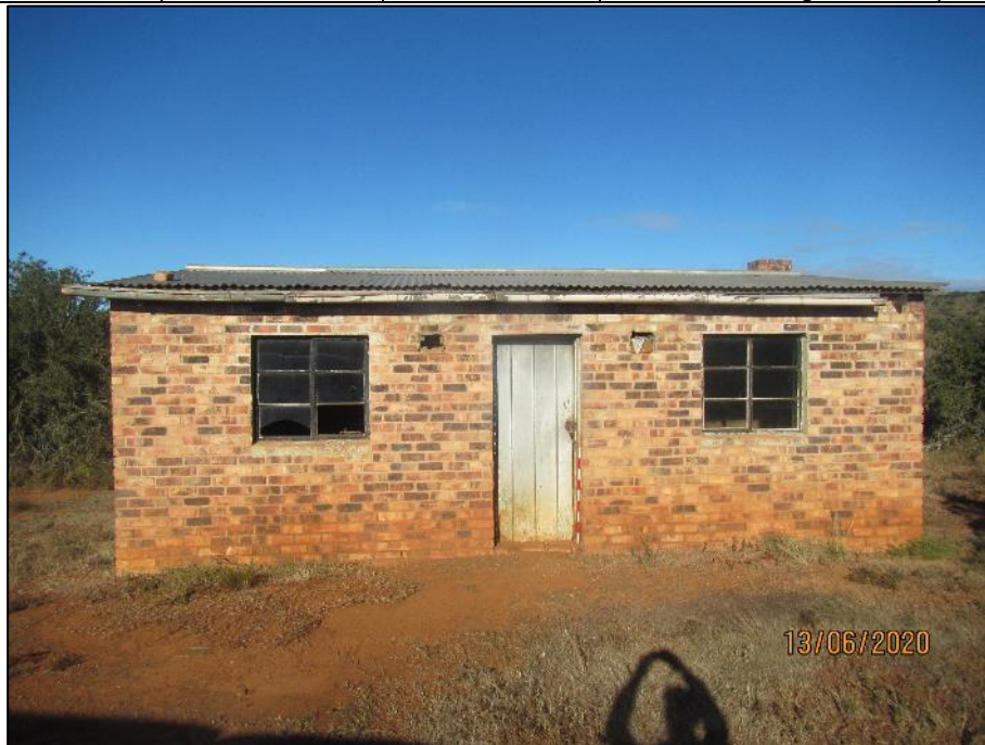
Figure 26 - View of the north-eastern facade
