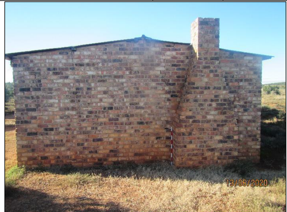
Figure 27 - View of the south-western facade
