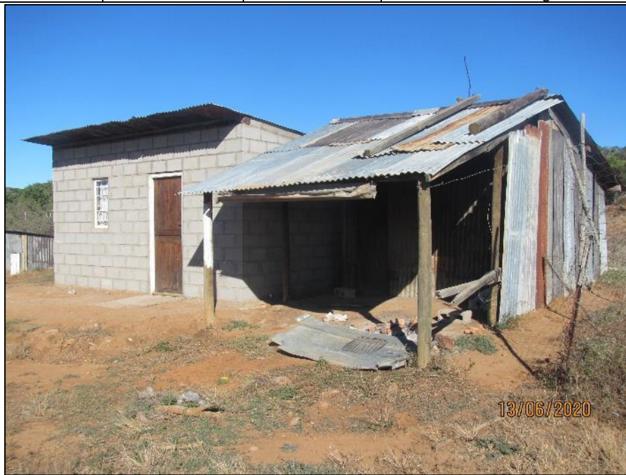
Figure 30 - View of the labourer house
