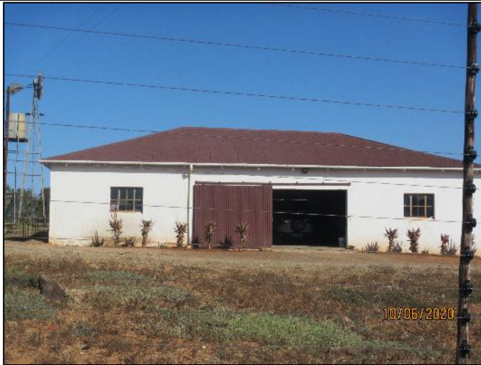
Figure 53 - View of the garage next to the house.
