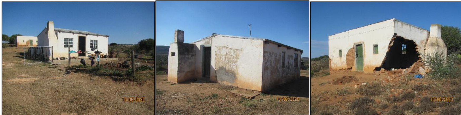
Figure 57 - View of the three labourer houses at WWF4-09.
