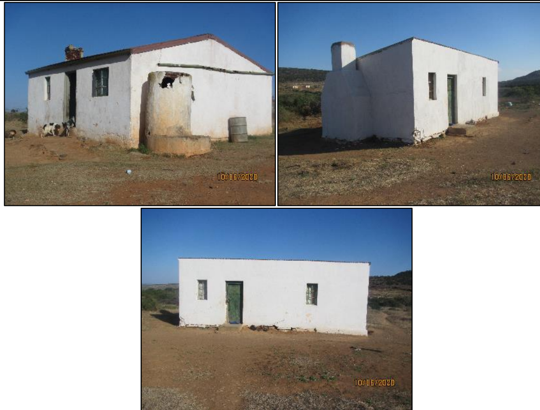
Figure 68 - View of the labourer houses at WWF4-13.
