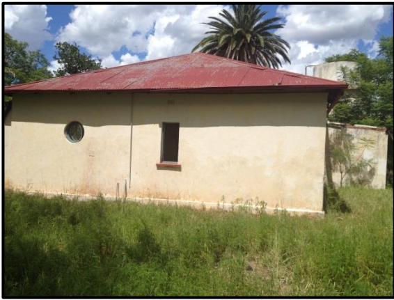
Figure 12: Structures on site 1
