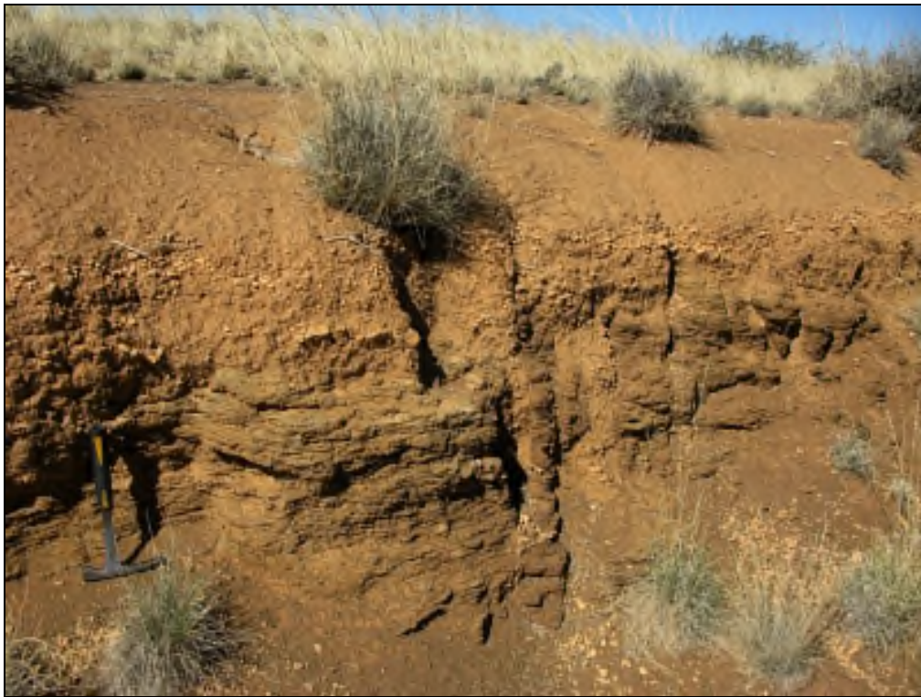
Fig. 33a. Deeply-weathered dolerite sabunga overlain by silty alluvial soils with nodular calcrete horizon, borrow pit on Kopjes Vley 281 (Loc. 040) (Hammer = 30 cm).
