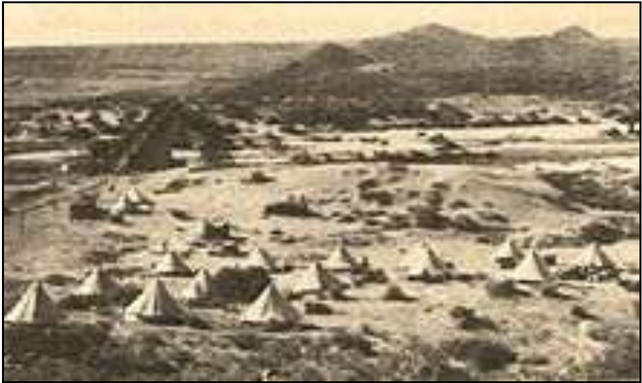
Figure 8 - A picture showing a construction camp of a railway line in the Karoo by the Cape Government Railways in 1870s.
