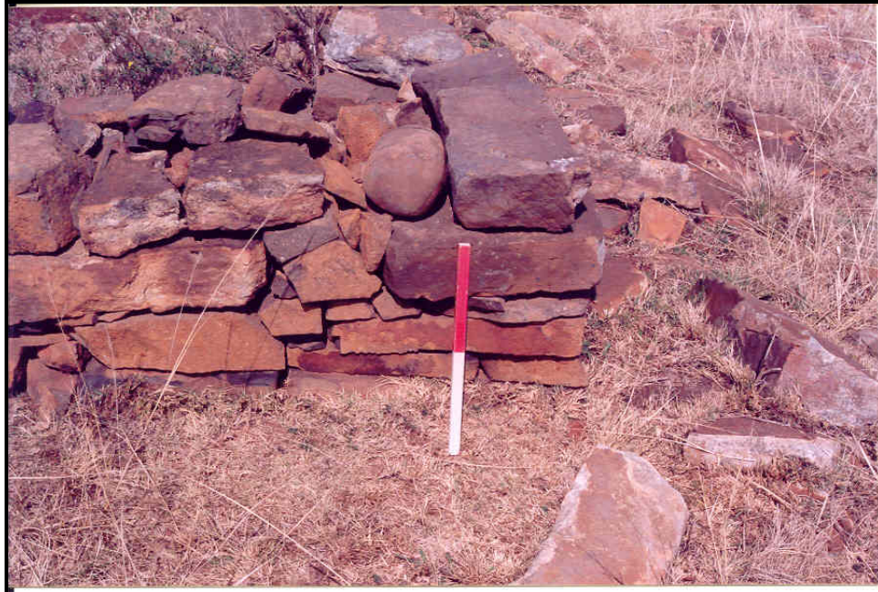
Figure 29 – Stone work on main house
