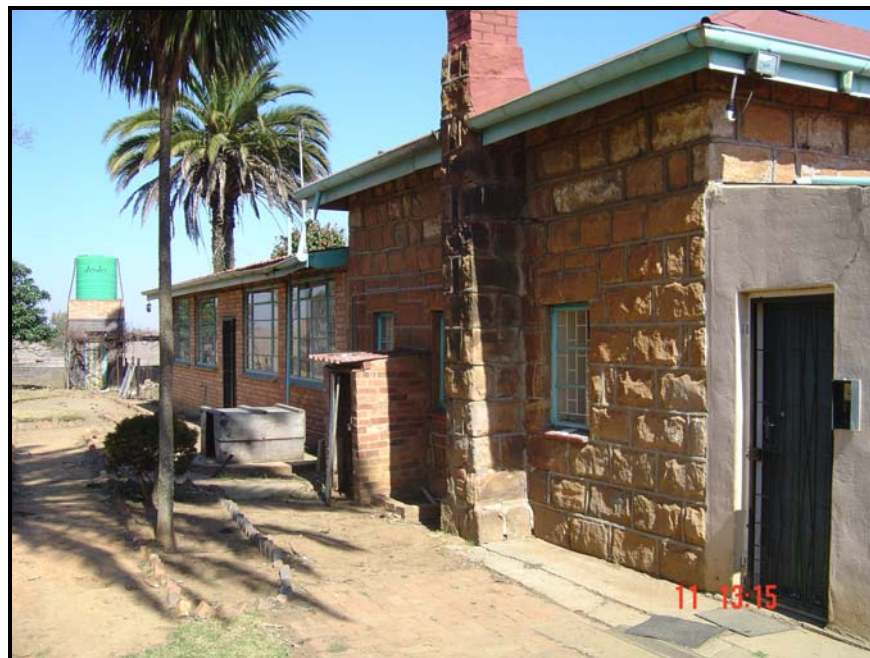
Figure 5 – Addition to original house
