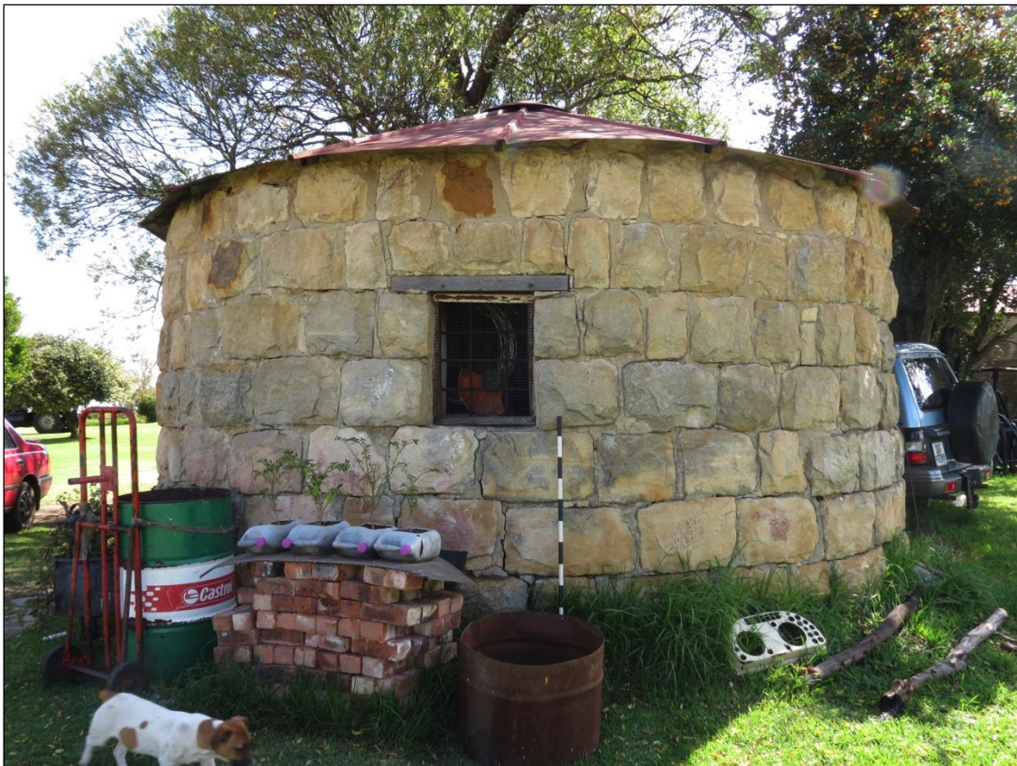
Figure 27—Another view of the rondavel structure. Note the small rectangular window with wooden frame and lintel.
