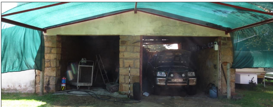
Figure 28–General view of the structure.
