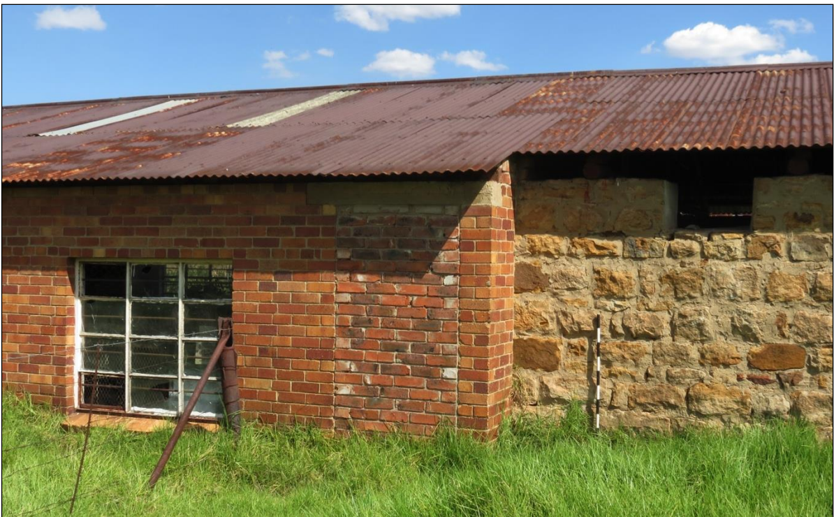
Figure 30—Different phases in the construction and use of the building can be seen from this image. The brick sections on the left would have represented a second or potentially third building phase with the sandstone component on the right potentially younger than the sandstone section on the south-eastern end of the site.
