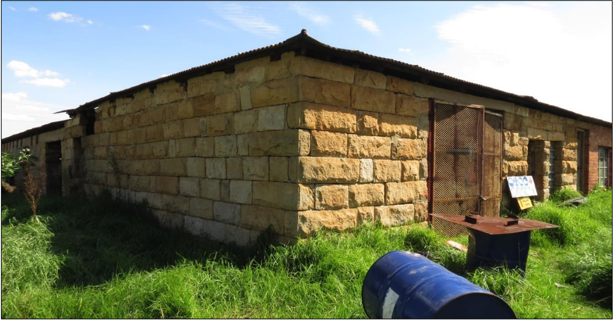
Figure 29—The south-eastern corner of the building representing what appears to be the oldest component of the site. Sandstone lintels above the window and door openings can be seen on the right.
