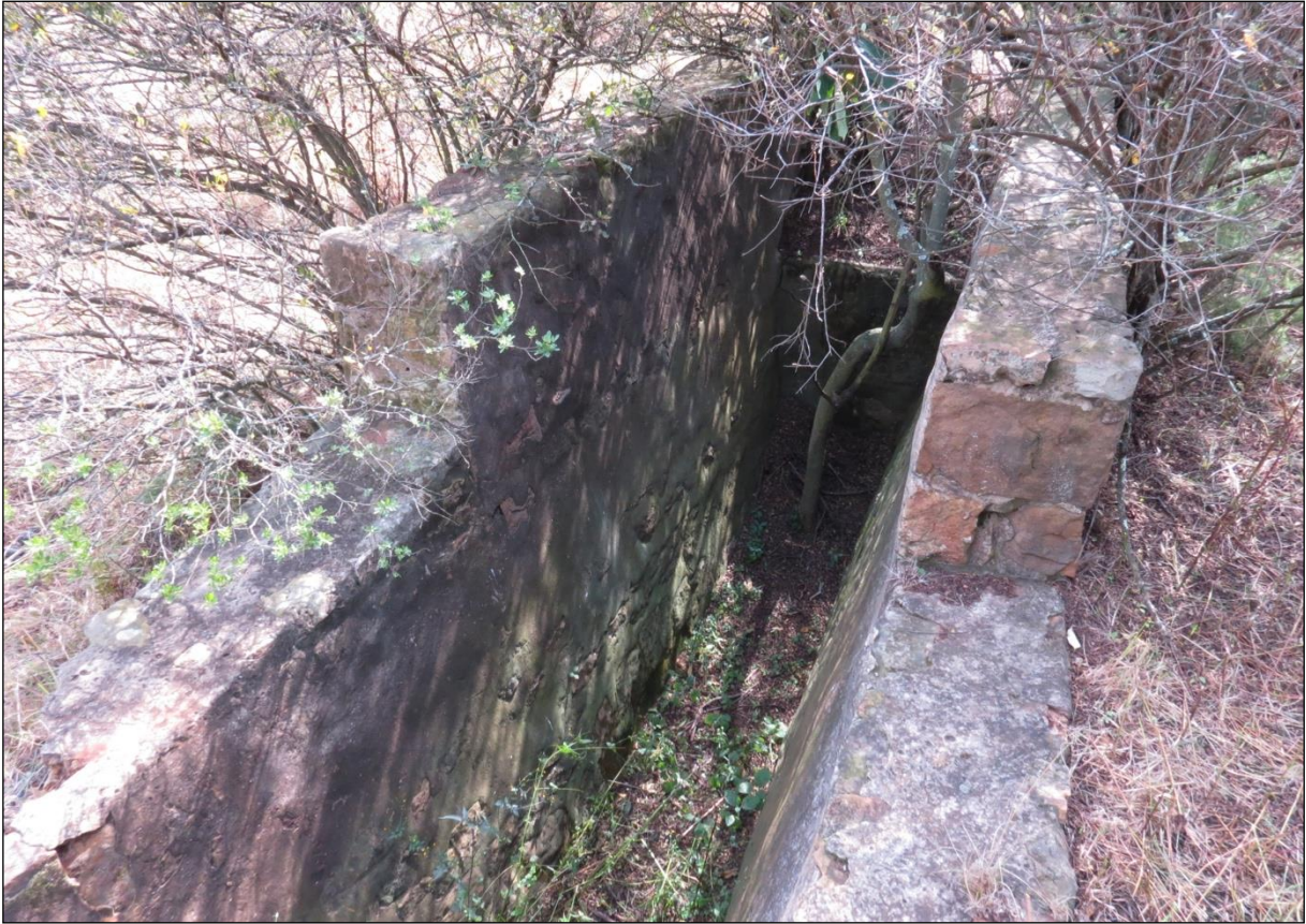
Figure 18 –General view of a section of the dipping structure. The vegetation already well established within the structure provides some indication of its age.
