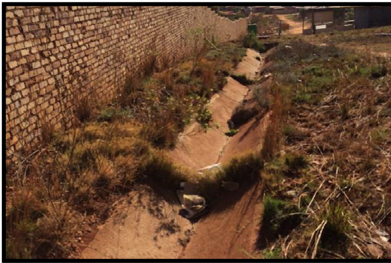
Figure 9: Existing Stormwater Channel
