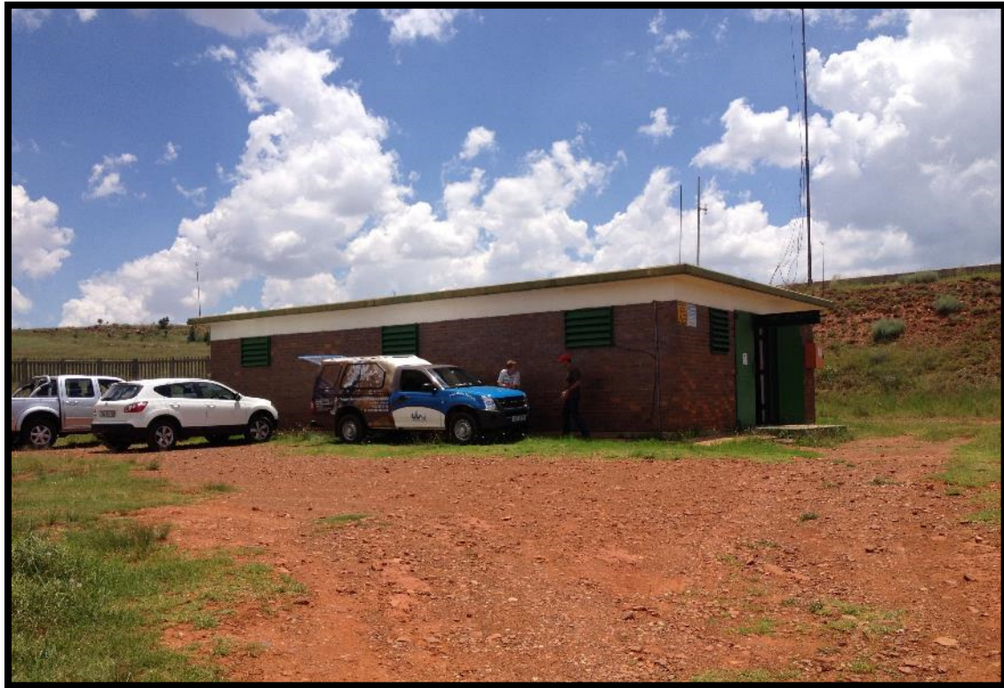
Figure 15: Existing pump station at Hospital Hill Reservoir
