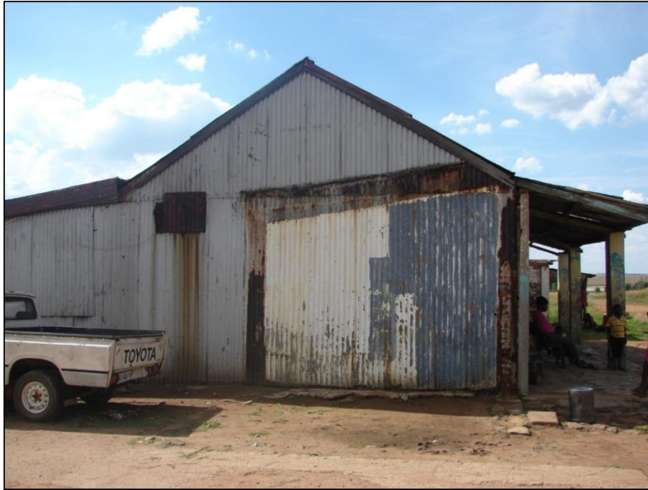
Figure 46 - Left, south, façade of the shop built from Corrugated Iron Sheets, note the veranda on the right end of the picture and the back extension to the left end of the picture. © Tomose @ PGS.
