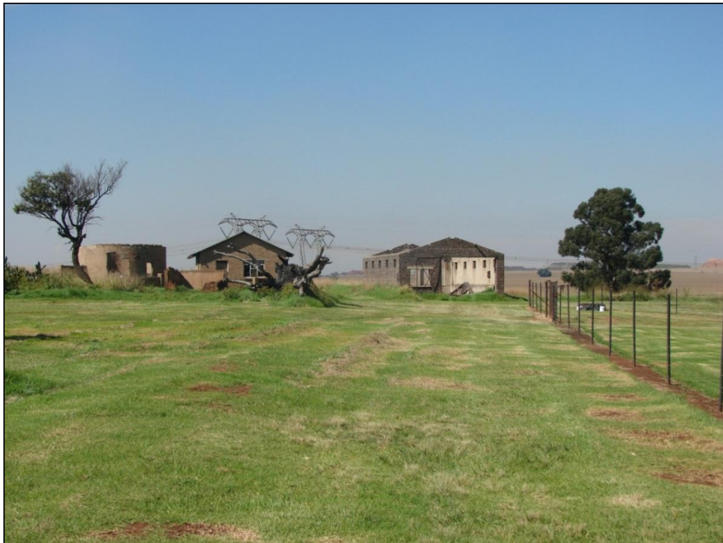
Figure 26 - Dilapidated roundavel, small square structure in front, a modern cottage & dilapidated old shed in fabricated brick- no roof, windows, and door. ©Tomose @ PGS
