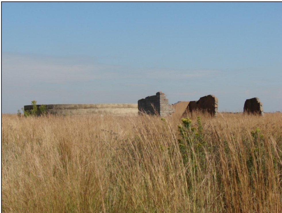
Figure 22 - Structure No.2 and reservoir. ©Tomose @ PGS
