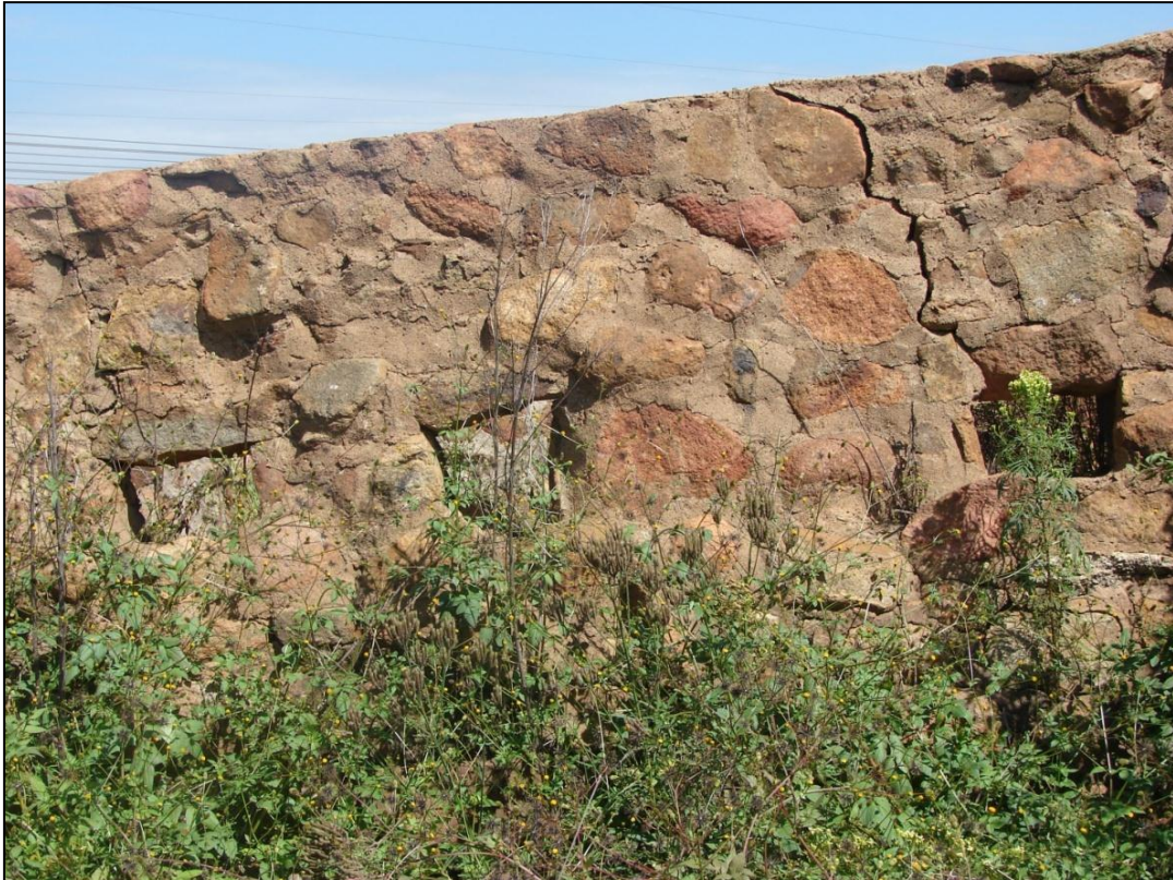
Figure 29 -Stone and mortar kraal, note small window openings on the side of the kraal wall. © Tomose @ PGS
