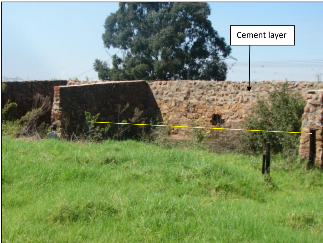
Figure 30 - Cement layer, north face of the kraal. Note the window opening; stones have fall on the window.
