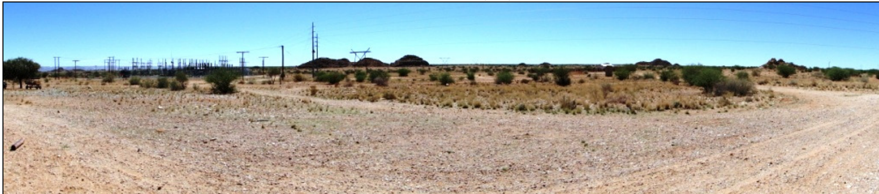
Photo 10: Perspective shows Skuitdrift Sub- Station on the left hand side of the image and rocky hill bordering the site.
