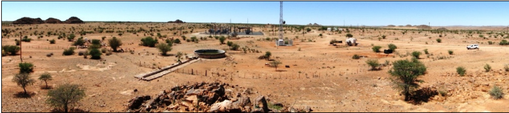
Photo 1: Panoramic perspective showing Skuitdrift Sub-Station adjacent to Skuitdrift outbuilding and dam.
