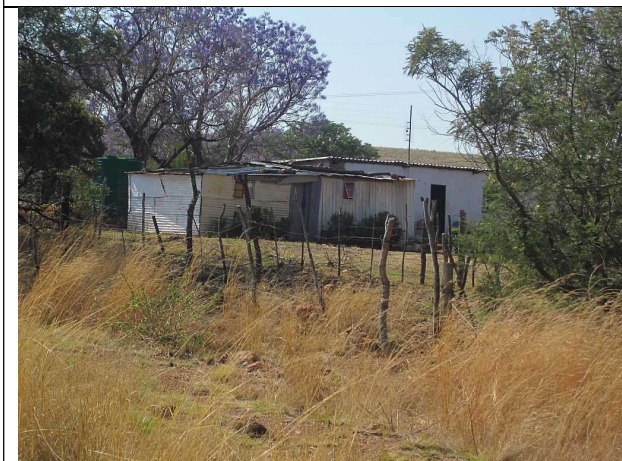
Figure 28. Corrugated add on structures at Feature 4
