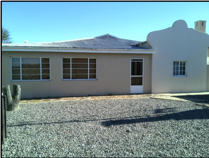
Figure 10: Farmhouse at Site 3.
