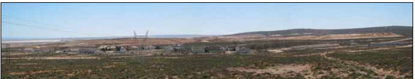
Figure 31: View towards the northwest over the old workers' compound, north of Kleinzee. The large power lines are relatively recent additions to the mining landscape.
