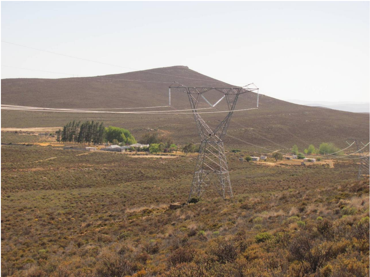
Figure 12 Existing 400 kV transmission lines cross the landscape close to Ou mure
