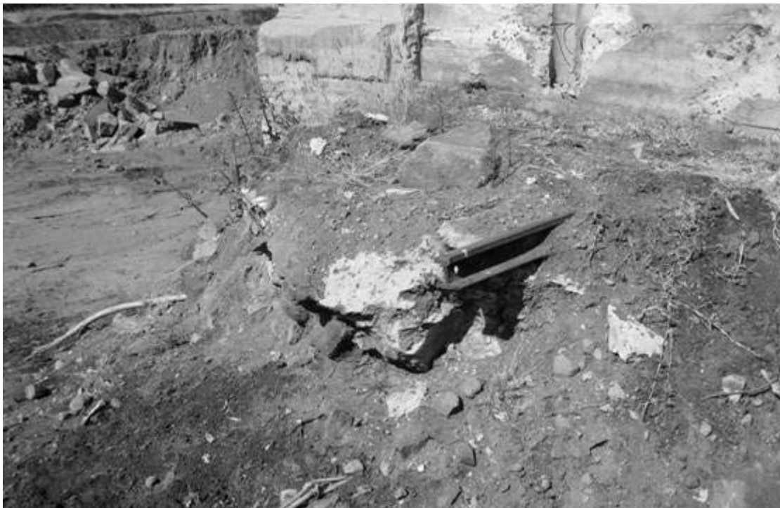
Figure 3. Remains of the rail on which coco pans retrieved ore from the mine headgear anchor block. The type of rail used is YSCOR steel from 1960's
