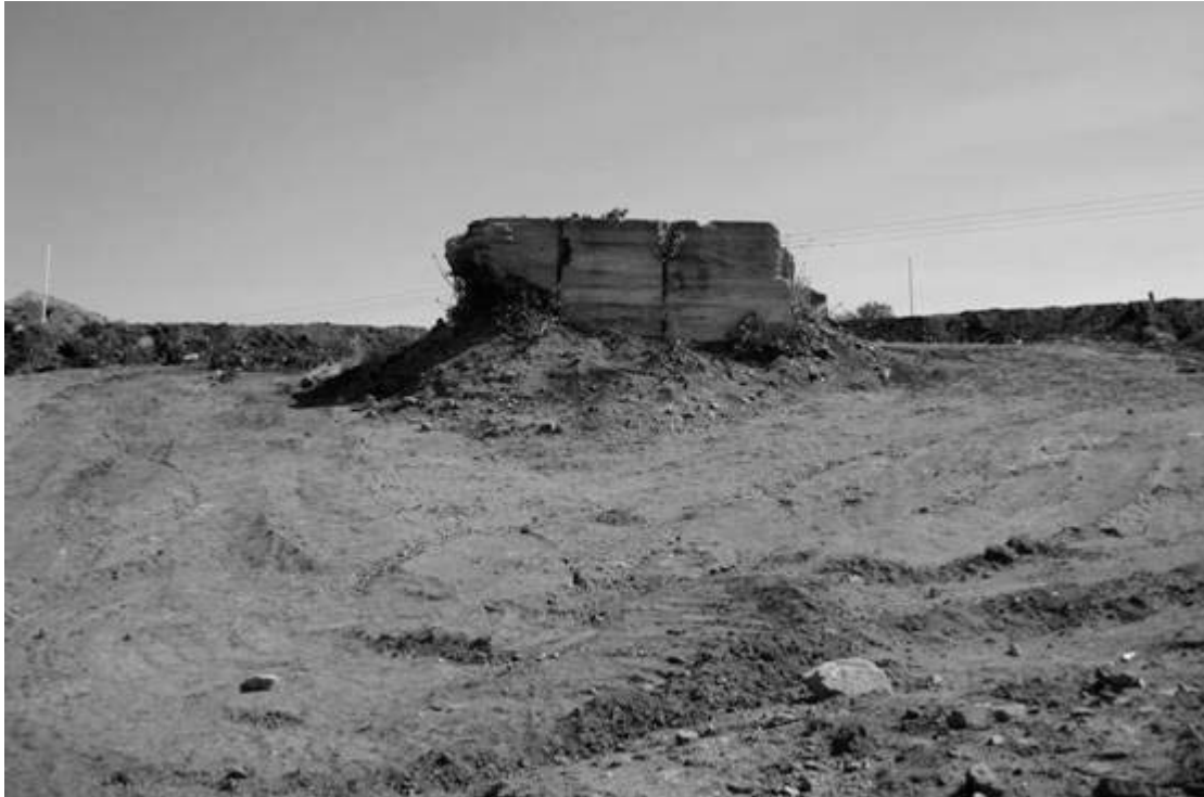
Figure 2. Remains of the headgear anchor block.
