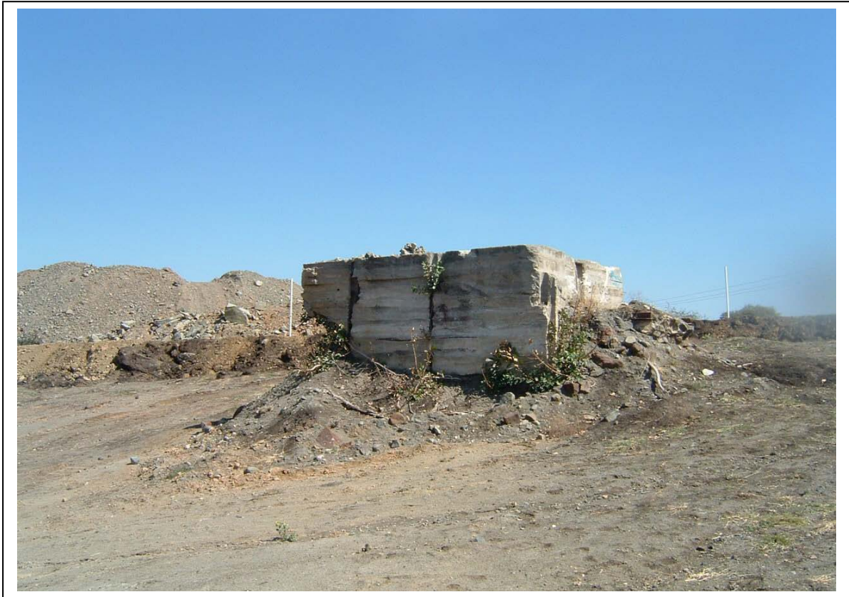
Figures 10 & 11- The anchor concrete block on which the mine's head gear rested (below), this is the most pronounced feature to be associated with the chrome mine (above). Pulleys with cables hoisted coco pans from the underground mine to the surface where the chrome ore was stock-piled (above).
