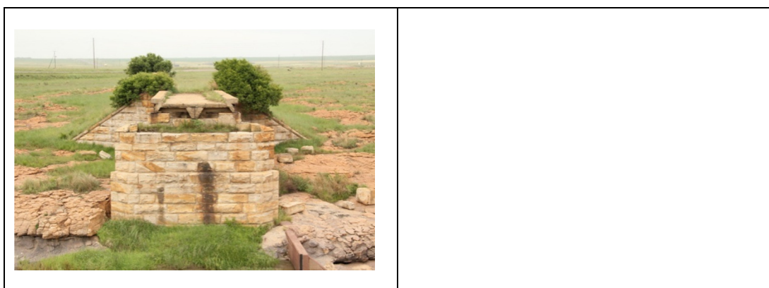
Fig. 7. Remains of an old sandstone bridge
