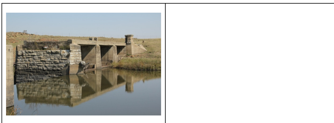
Fig. 7. An old bridge across the Leeuspuit.
