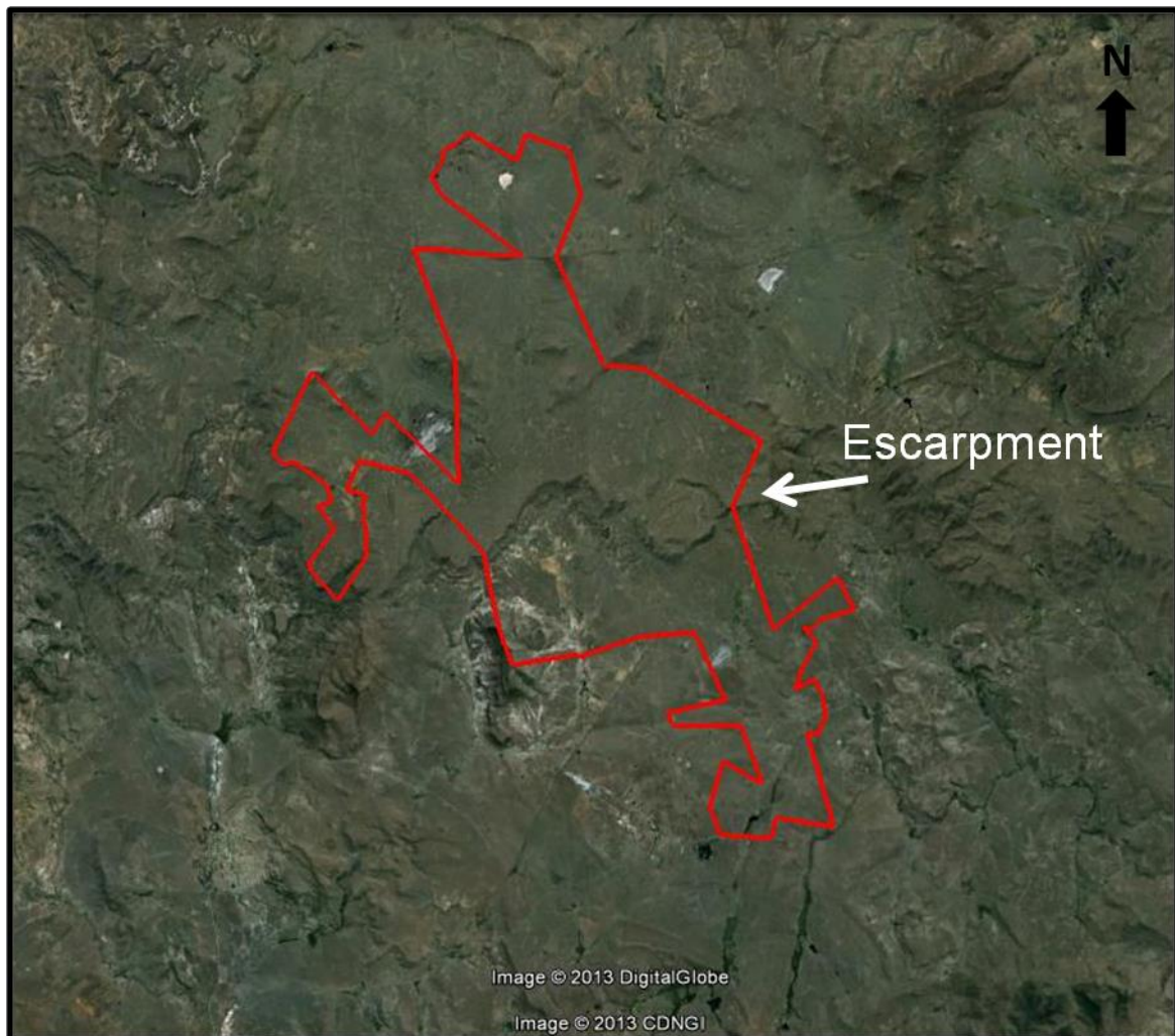
Figure 7: Google Earth image of the project area (the red polygon) and its environs. It is evident from the image that the project area is divided into northern and southern portions by an escarpment. The areas lying to the north and west of the escarpment are plains, with the southern area lying at lower altitudes. There are no signs of cultivation evident from the image and as such it is probable that the area is utilised for grazing and/or game farming.
