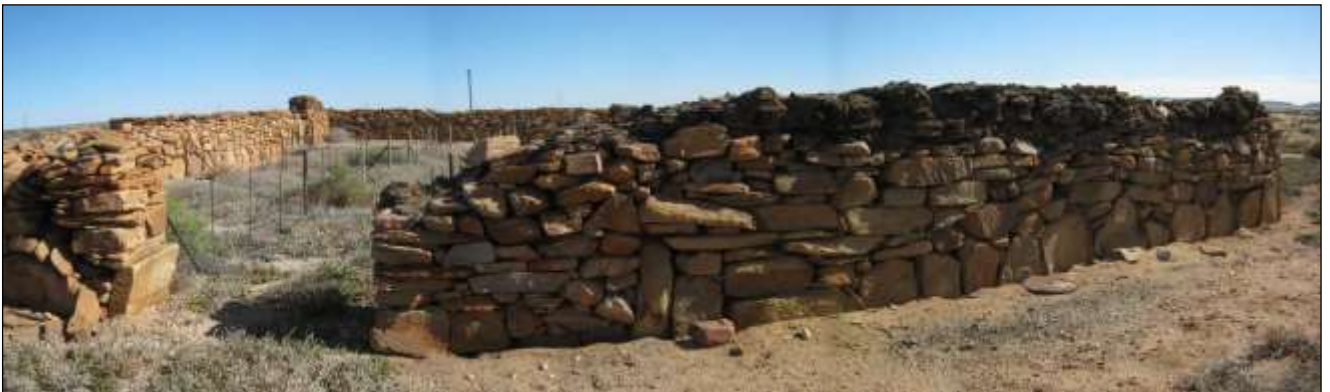
Figure 13: The stone kraal with dung on top of the walls at Poortjie.
