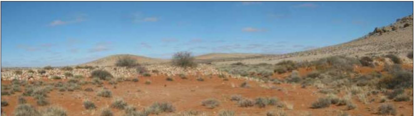
Figure 14: Earth dam with stone lining on the inner wall in the “poort” of Poortjie.
