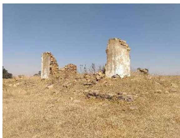
Remains of main structure at HST-001
