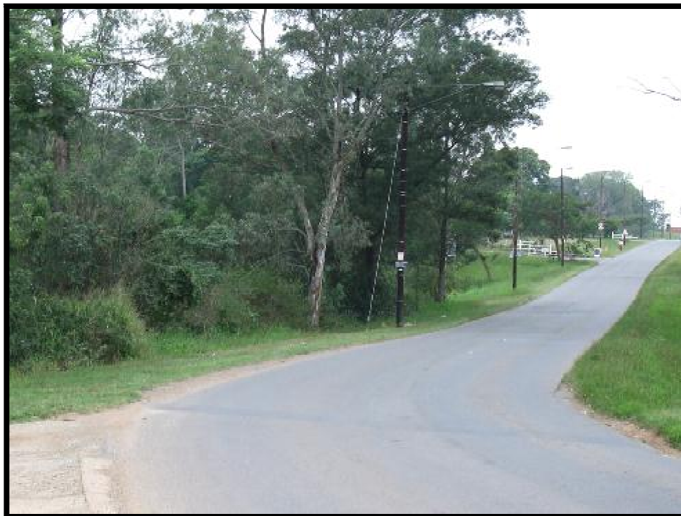
Figure 4. Start of Hesketh Drive Extension, Hayfields.
