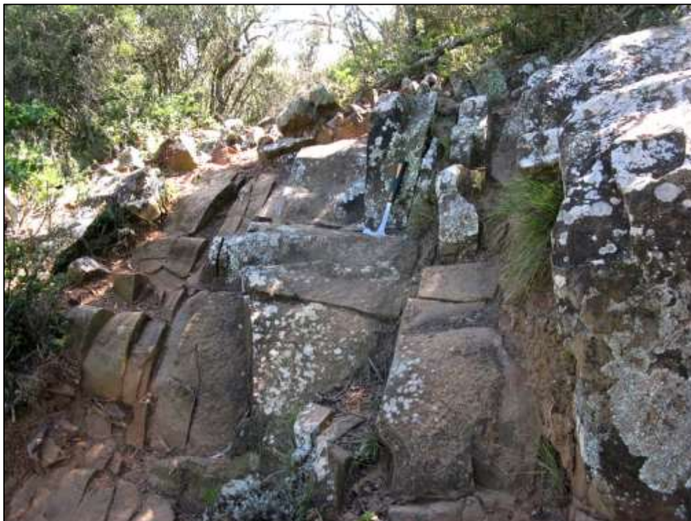
Fig. 12. Well-jointed brownish-weathering wackes of the Hexrivier Formation, Grassridge 187 (Loc. 659) (Hammer = 30 cm).
