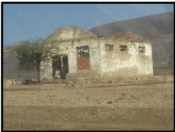
Figure 12. Trading Store 1. This building is damaged by fire and has been absconded.
