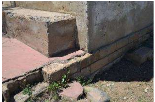
Mud-block construction.
