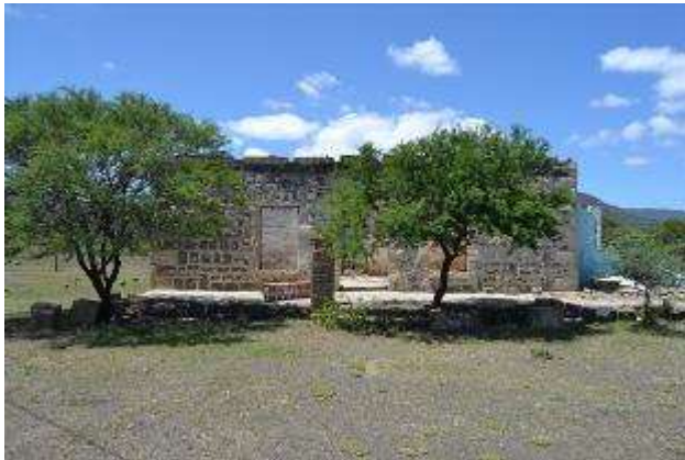
West facade (facing R33).
