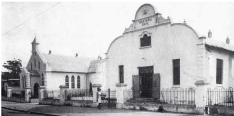
The Volkskool in Banhoek Road, Stellenbosch was demolished and the Volkskerk is now used by the Church of England.
