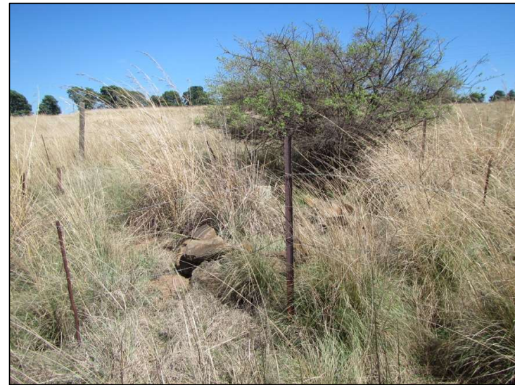
Figure 53 - Dilapidated fencing surrounding 023
