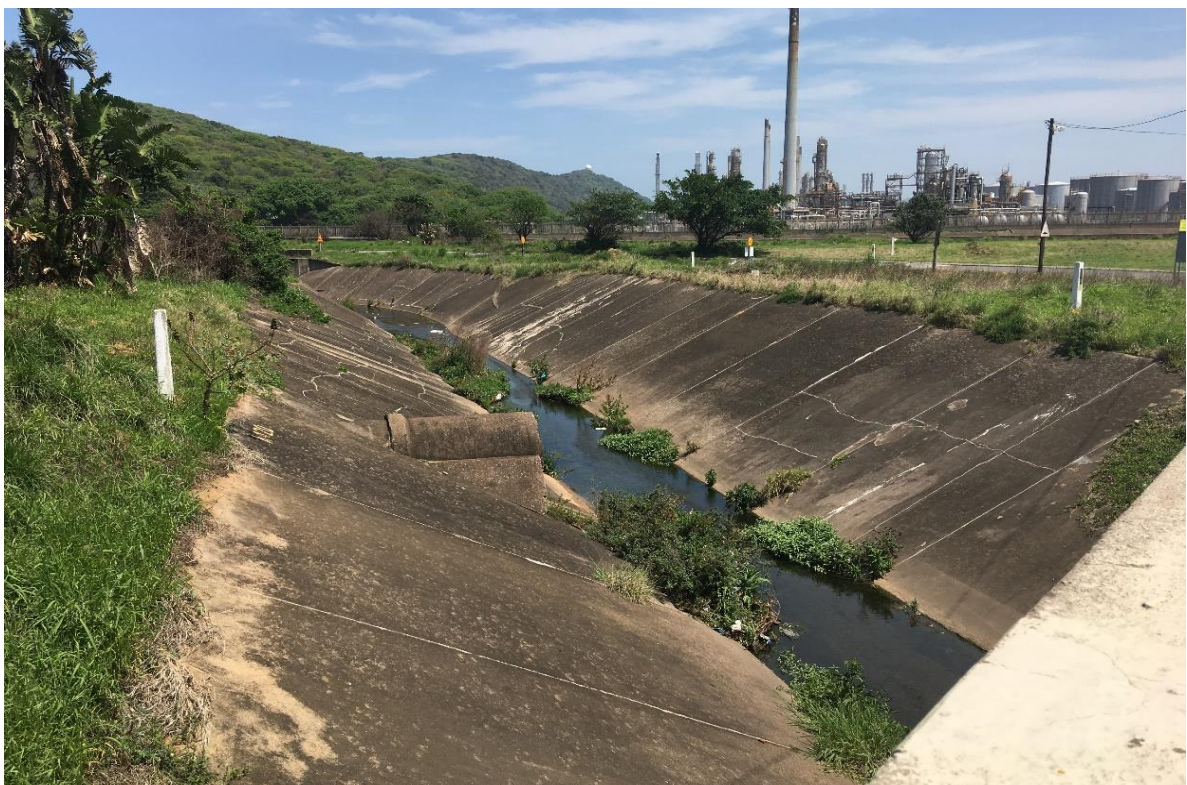
Figure 15: View across canal towards Engen refinery along Badulla Drive
