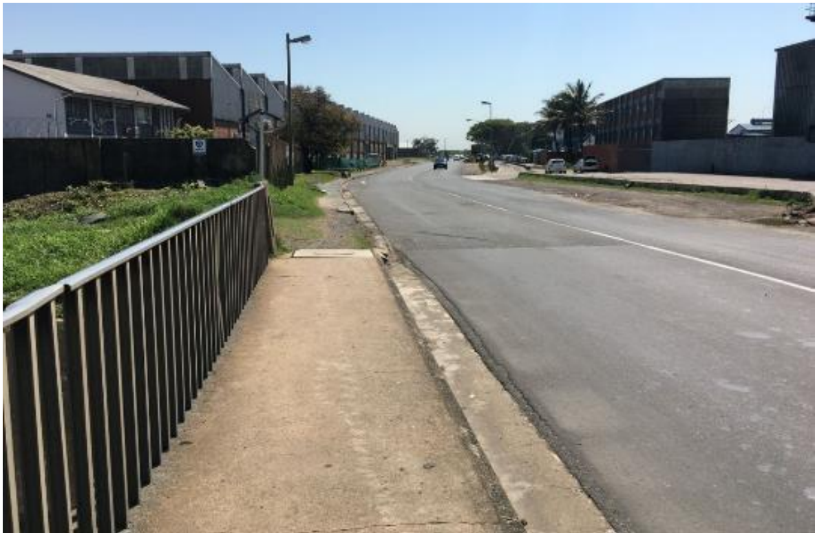
Figure 11: View of Joyner Road / Isipingo River canal crossing looking north-easterly
