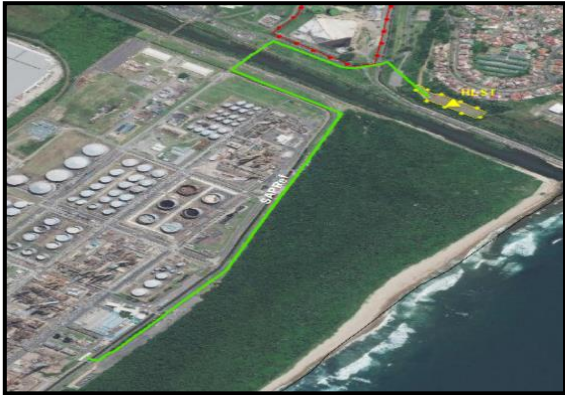
Figure 2: New pipeline to SAPREF
