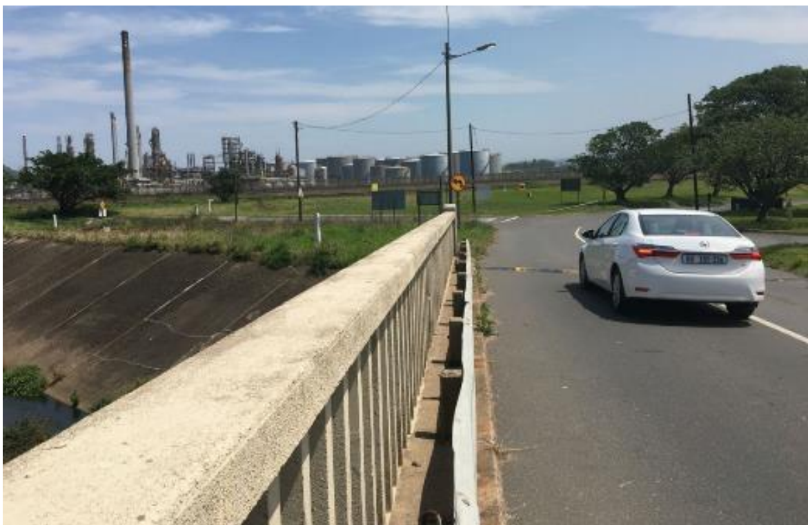
Figure 3: Travancore Drive crossing canal looking towards SAPREF
