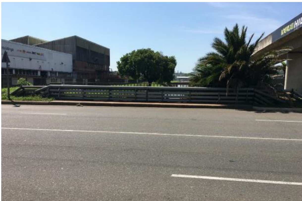
Figure 10: View of existing pipeline rack along R102 crossing Isipingo canal
