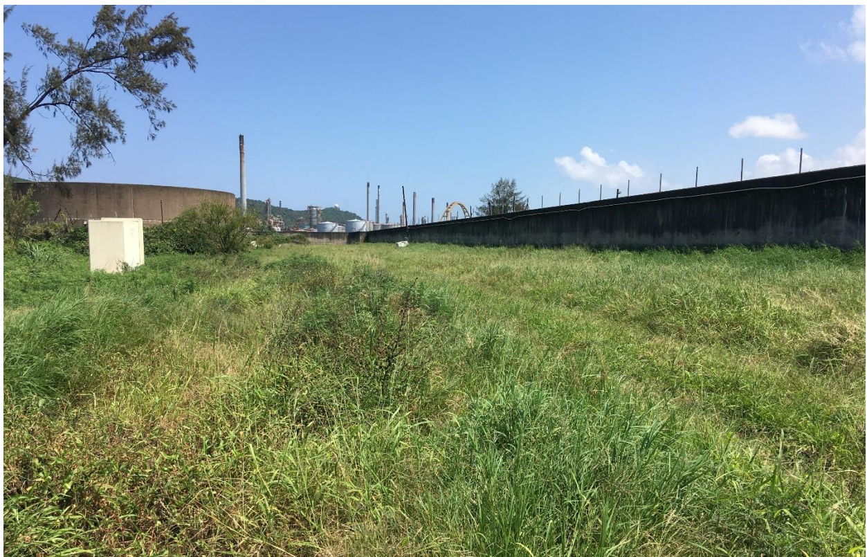
Figure 5: View along pipeline route along SAPREF boundary
