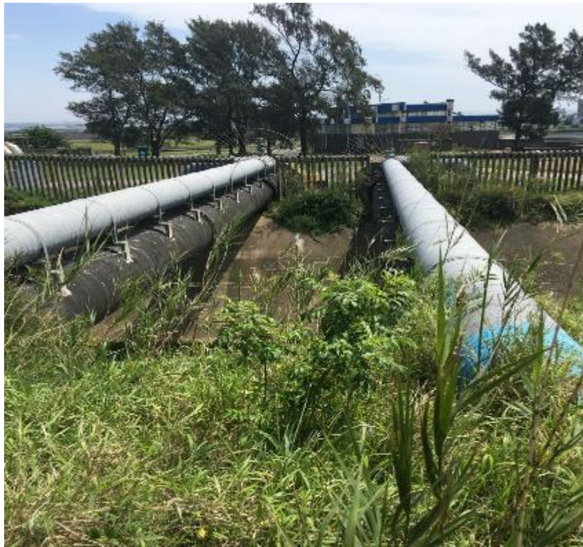
Figure 4: Pipelines crossing tributary canal with southern WWTW in background
